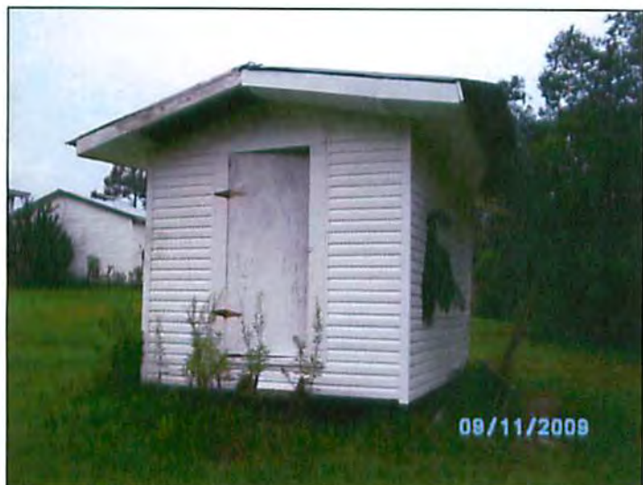
Yard Building/Pump House
