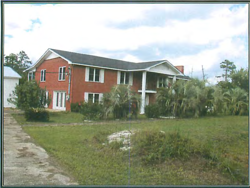
View of the southern side of the single family residence
