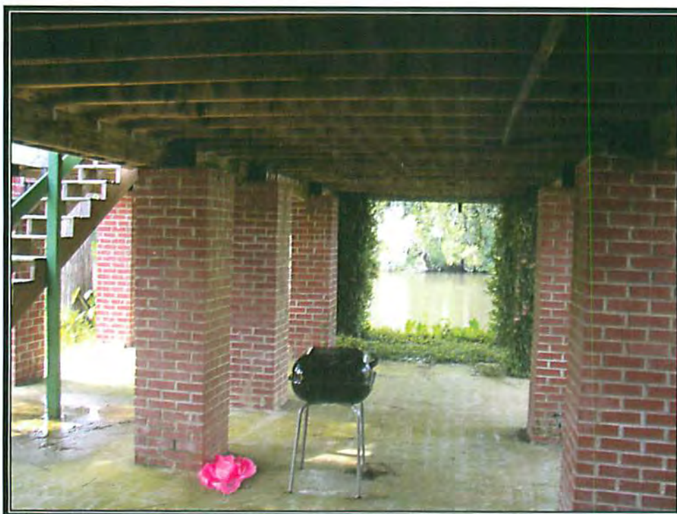
View of the area underneath the rear deck
