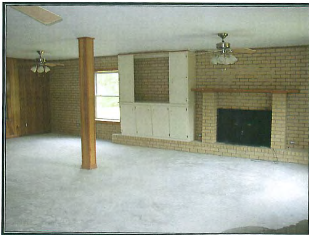
View of a family room (1 st Floor)
