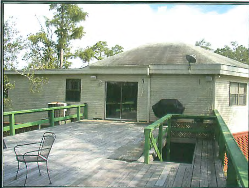
View of the northern side of the improvement facing south from rear deck
