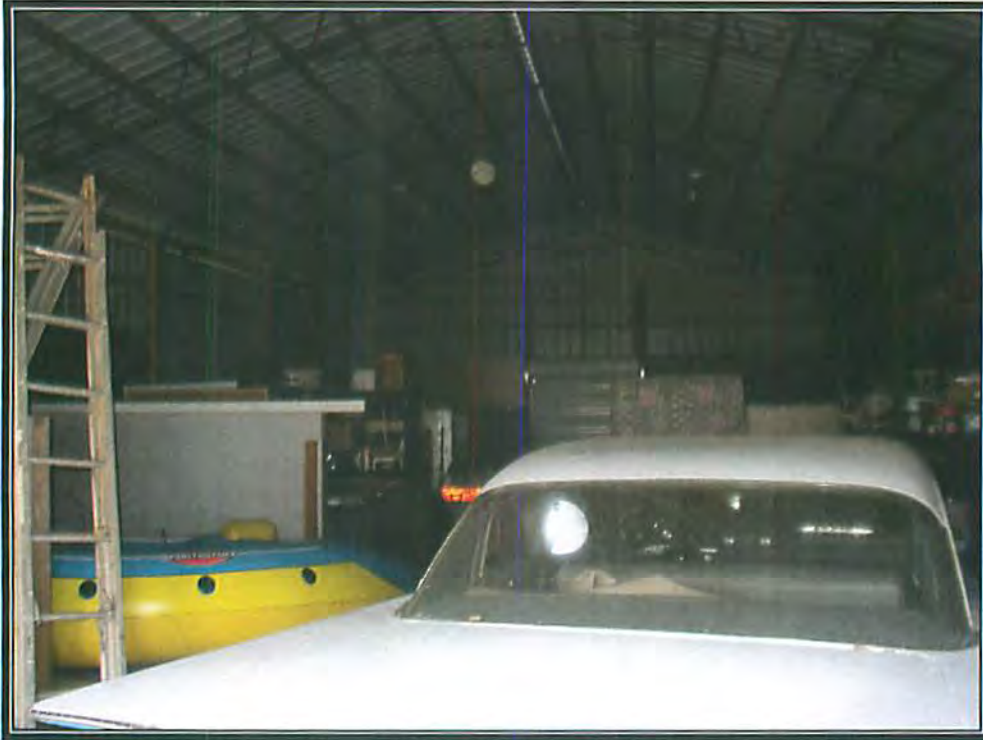
Interior view of the additional building identified as Building 2
