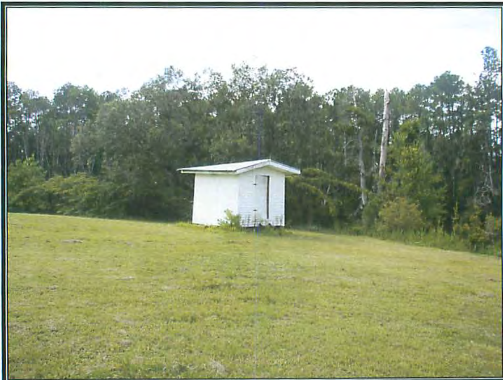
View of the well house that contains an artesian well, and houses the pump that pulls water from the Perdido River to operate the fountains in the pond
