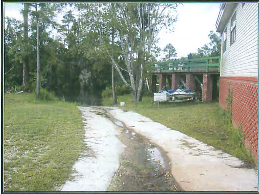
View of the concrete boat ramp as it extends along the western side of the improvement and terminates into the Perdido River
