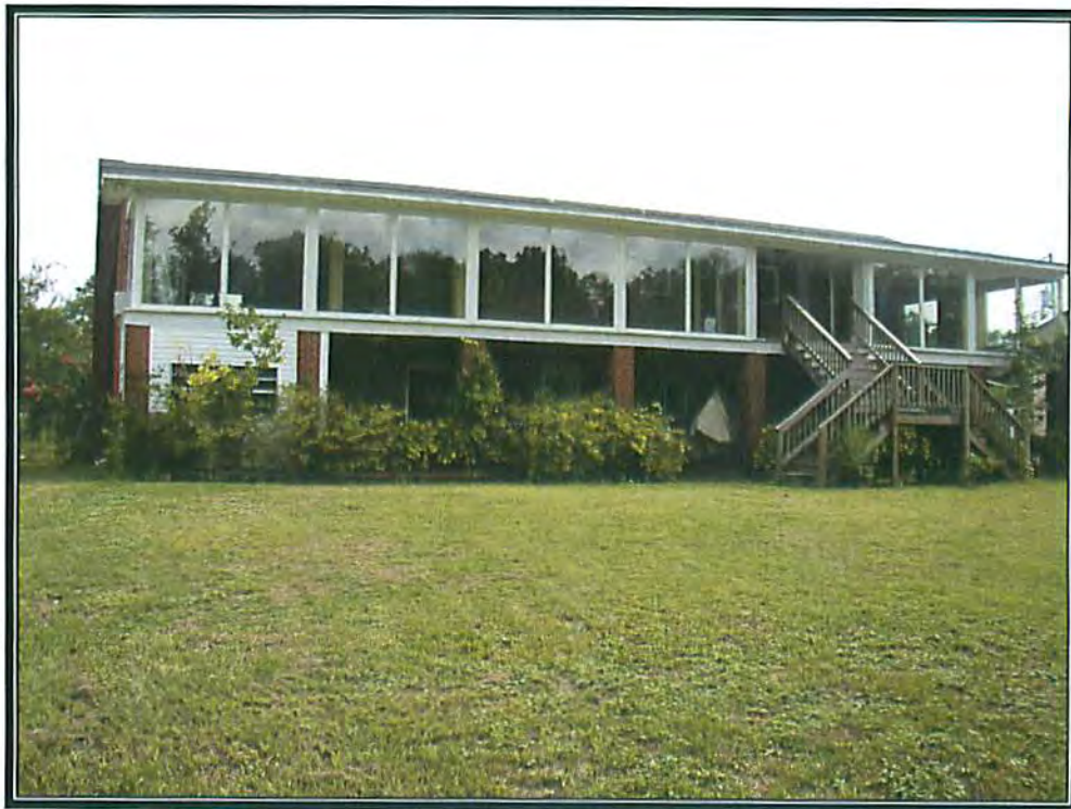
View of the northern side of the single family residence facing south
